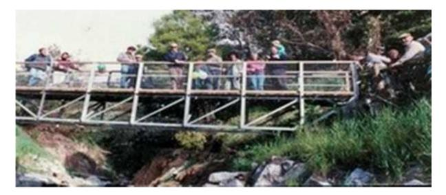
As a result of serious floods in December 1988, the foundations of the bridge on the east bank were almost completely washed away. Fortunately they were able to be repaired before the bridge collapsed. The photo shows the seriousness of the flood damage to the bridge.
