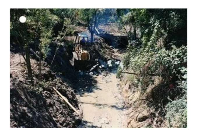
At the site, between Whale Rock and Grange bridge, where the bottom and banks had been severely eroded, the engineers built the bed up with half a meter of granite boulders as well as lining the banks particularly on the west side.
