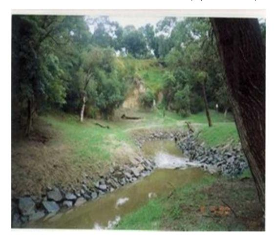
As part of this project, Melbourne Water kindly rebuilt some 15 meters of the east bank of the Granites which, over the years had been badly eroded by the stream when in flood.
