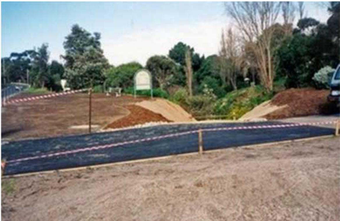
The floodway was cut in, the top area and the banks graded & the floodway provided with a road metal base and a granitic sand surface. While really designed as a floodway, it makes an excellent track.
